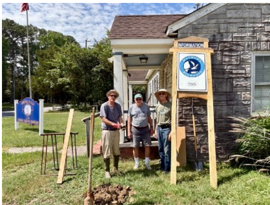
Mike Moore, Pete Hall, Philip Mutton installing the kiosk
